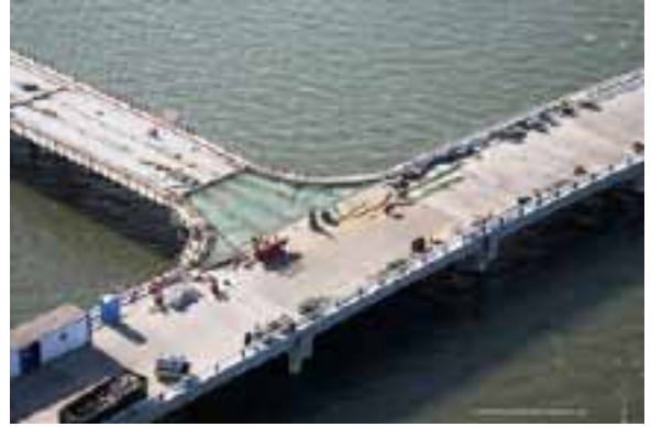
Framing at the intersection of the mainline and connector bridges.
