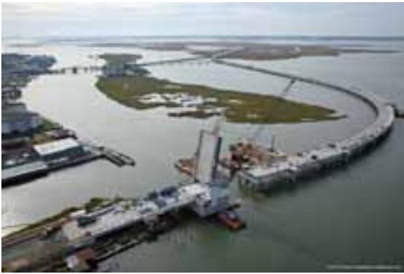
The new Chincoteague Island Bridge.
