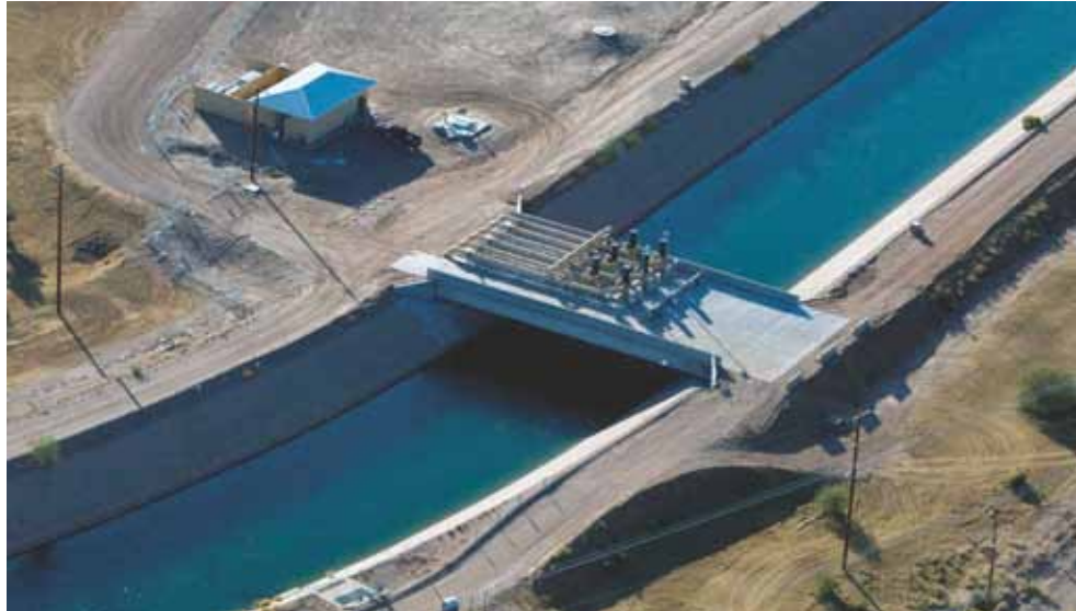
Aerial view of the bridge-mounted pumping station. All photos: Central Arizona Project/Central Arizona Water Conservation District.
