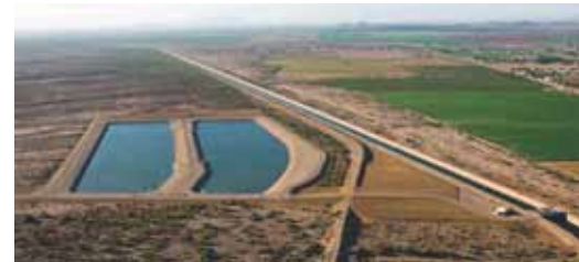
Aerial view of canal, recharge basins, and the pumping station.
