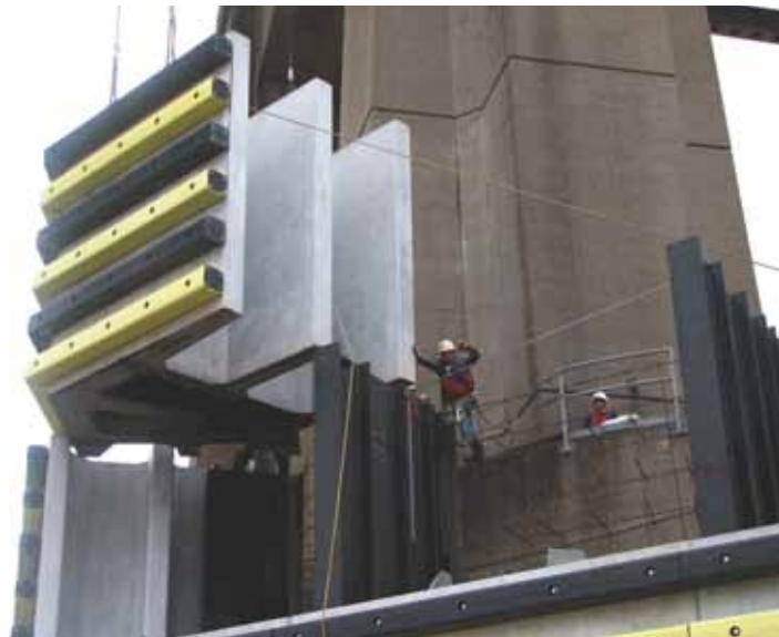
A corner module being slid into place for the Pier 5 fender.
