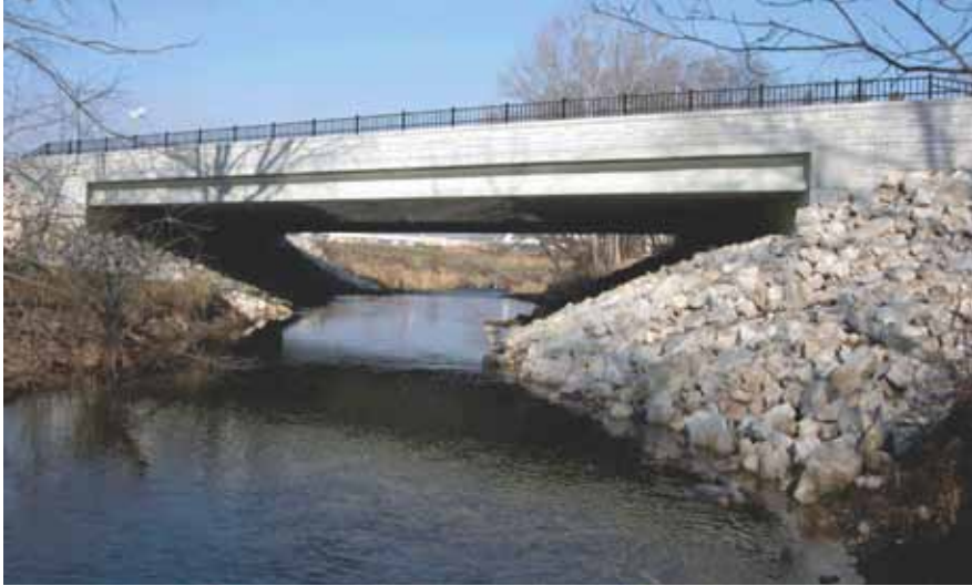
The nearly completed West Pioneer Road Bridge spans the East Branch Fond du Lac River. When weather warms, the contractor will stain the formed stone finish to replicate the limestone rock found in the area. Photo: Paul Sponholz, Fond du Lac County, Wis.
