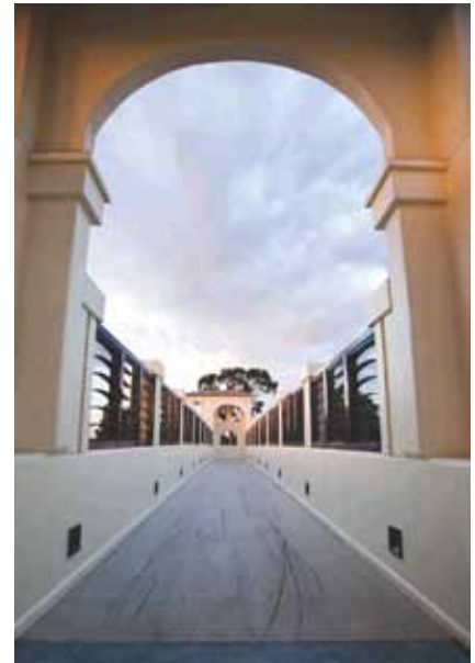
The girders also act as the parapet walls along the walkway of the bridge. Photo: Paul Savage, Photographer.
