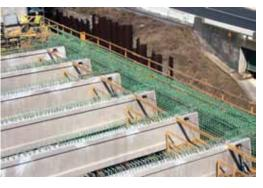
Precast, pretensioned and post-tensioned concrete floor beams are supported by the edge girders with reinforcement that extends from the beams into the girders. Photo: AECOM.
