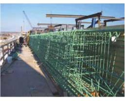
The use of epoxy-coated reinforcement throughout the structure along with several other anti-corrosion measures will help the new Indian River Inlet Bridge achieve a planned 100-year service life in the corrosive marine environment near the Atlantic Ocean. Photo: AECOM.
