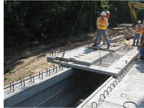
Placing and aligning precast, prestressed concrete overhang panels used on the Farm-to-Market Road 1885 Bridge over Rock Creek.
