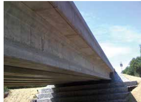
The underside view of the Farm-to-Market Road 1885 Bridge over Rock Creek near Cool, Tex., shows the use of the precast, prestressed concrete overhang panel system.
