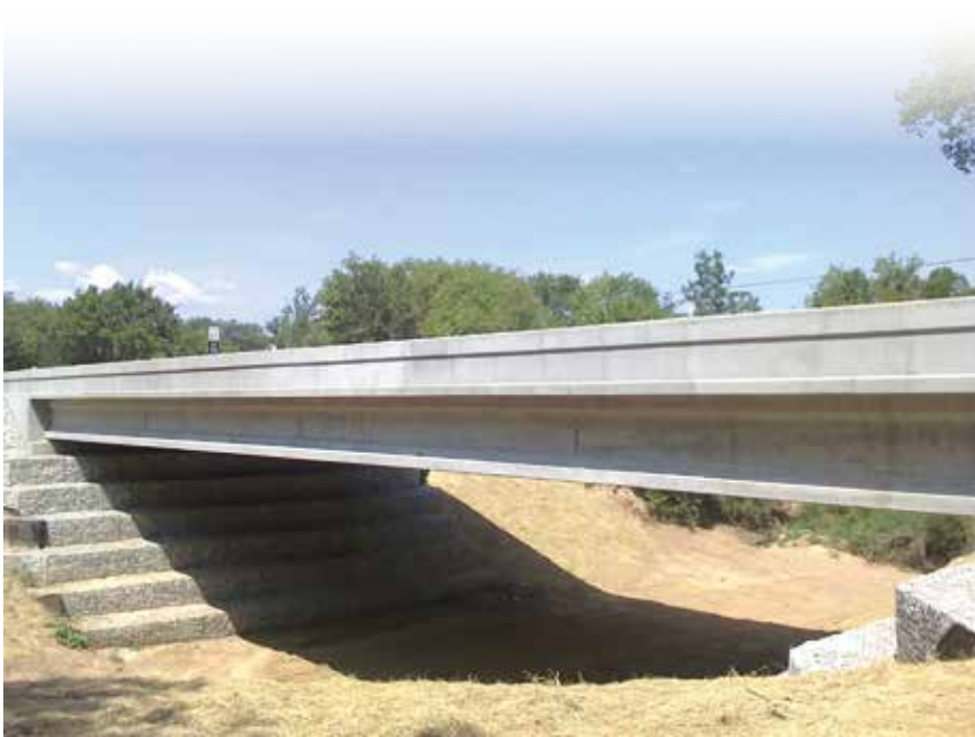
The completed Farm-to-Market Road 1885 Bridge over Rock Creek was the first bridge in Texas to use the precast, prestressed concrete overhang panel system. All photos: Texas Department of Transportation.
