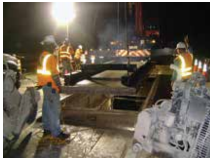
The existing I-75 deck was removed during a nighttime replacement operation.
