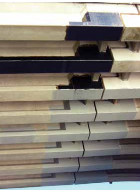
Carbon-fiber reinforced polymer hinge strengthening completed and painted with gray color UV protective coating.
