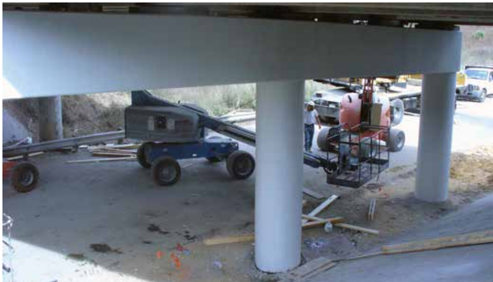
Another view of the repaired columns and pier caps that were part of the rehabilitation project for the Florida Turnpike over the SR 561 Bridge.
