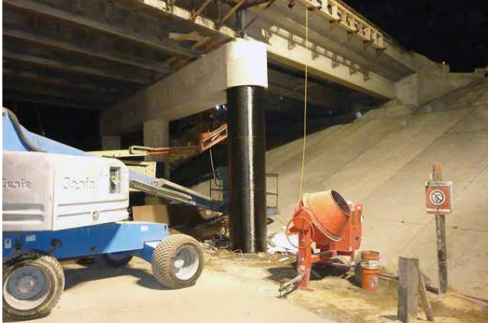
An example of column repairs for the Florida Turnpike over the SR 561 Bridge.
