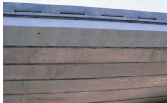
Completed box girders repairs.
