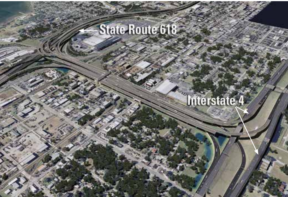
Rendering of the project that shows the completed Interstate 4/Selmon Expressway connector drawn into its location within an actual aerial photo. All photos: Florida Department of Transportation.
