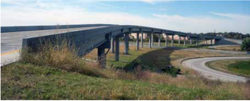
Precast concrete, curved Nebraska University (NU) girders carrying Interstate 470 eastbound connector road over U.S. 50 at Lee's Summit, Mo.
