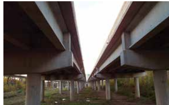
Precast concrete girder spans provide economy over floodplains in the Route 370 Missouri River Bridge at St. Charles, Mo.
