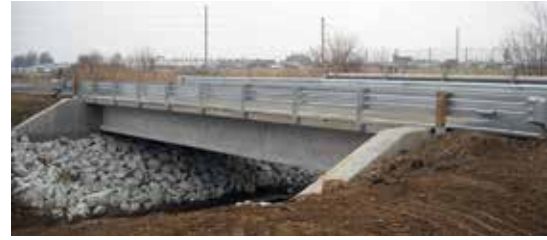
Designer led, design-build was used to construct multiple small bridges for the owner, ATK, in Independence, Mo., in the less than $1M category.
