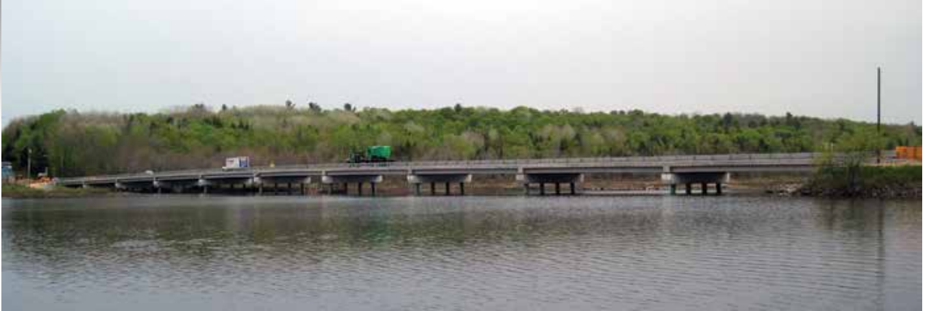
The 790-ft-long, two-lane bridge consists of ten 79-ft spans arranged in two 5-span continuous units spanning over a shallow pond. Photo: Lane Construction.
