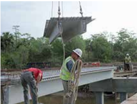
Typical precast prestressed modified Florida double tee being hoisted for placement.
