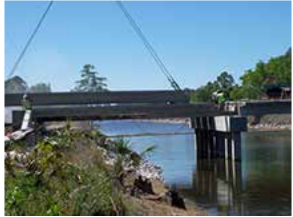
Beam installation between end bent No. 1 and intermediate bent No. 1.
