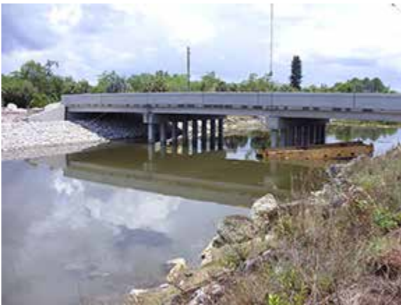
Profile view of bridge looking north.
