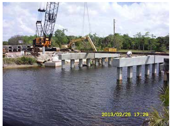
Final erection of intermediate bents — elastometric bearing pads being set.
