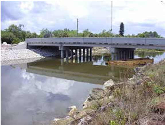
Profile view of bridge looking north.
