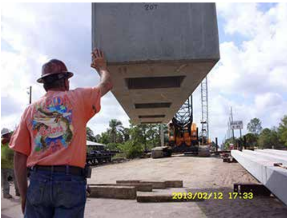
Precast pile cap being delivered to the site.
