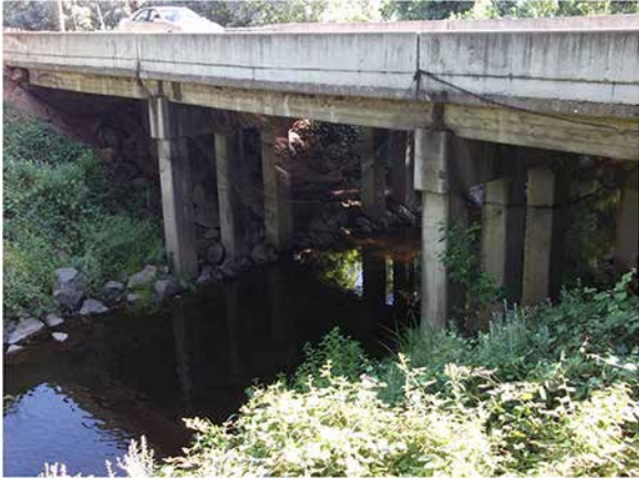
The old three-span Craig Creek Bridge that was replaced.
