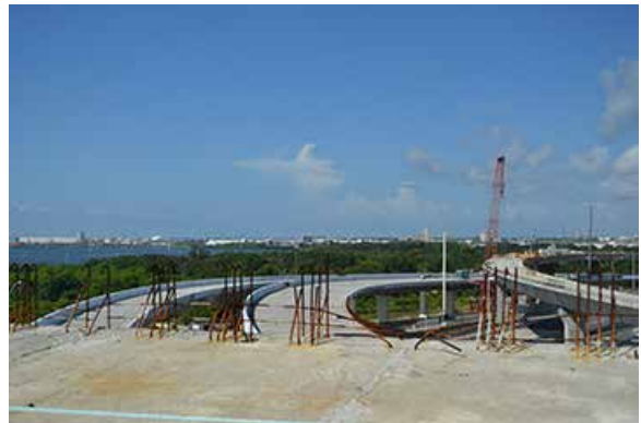
Segmental bridge construction with downtown Tampa in the background.
