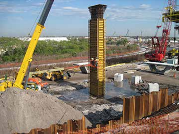
One of the project’s many columns constructed using “bottom-up” concrete placement.
