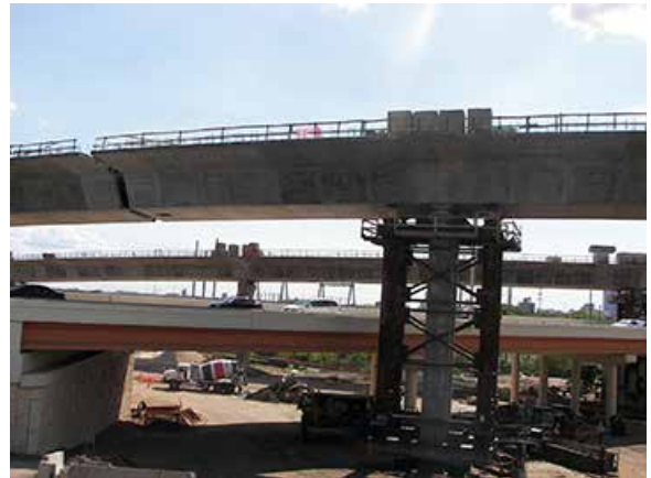
Segmental bridge construction over eastbound Interstate 4.
