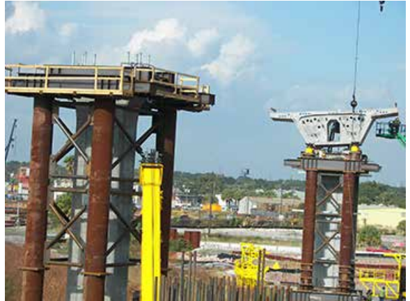
Crews place the project’s first pier segment in November 2010.
