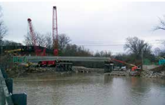
Erection of the precast concrete segments on temporary towers.
