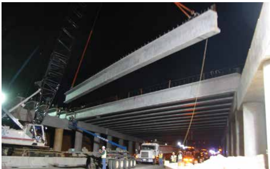
Georgia Department of Transportation achieved a 20% decrease in shipping weight using girders with a 10.0 ksi compressive strength lightweight concrete. Photo: Paul Liles, Georgia Department of Transportation.
