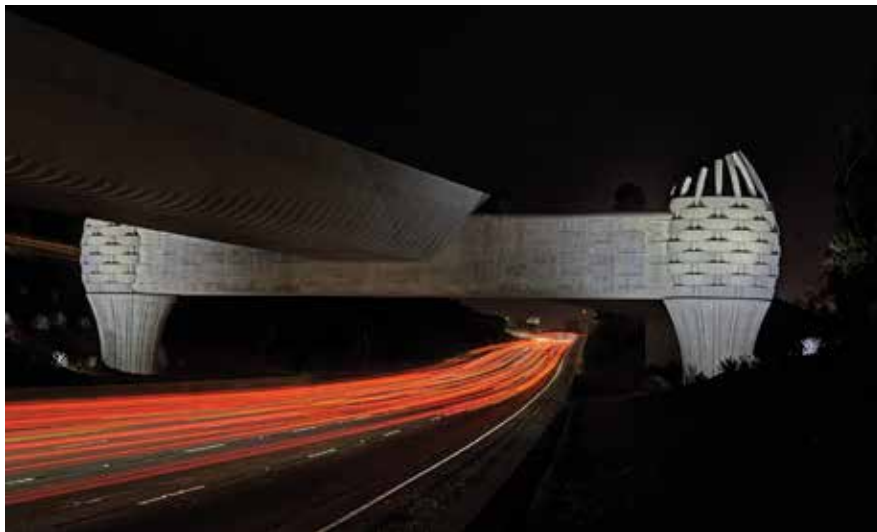
Lights wash the sides of the bridge at night, emphasizing the basket-like appearance of the column tops and the reed-like texture of the horizontal support.
