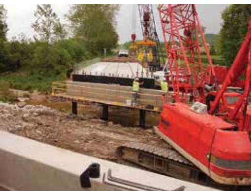
Setting adjacent beams.
