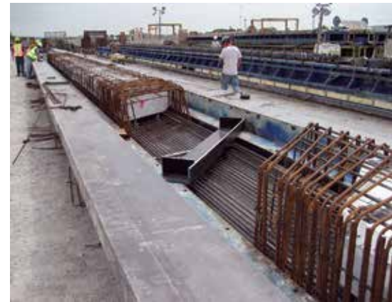
Prestressed concrete box beam fabrication.
