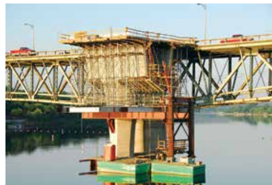
Pier table constructed on falsework.
