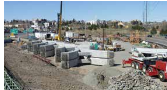
The precast concrete interior piers were cast and stored horizontally.
