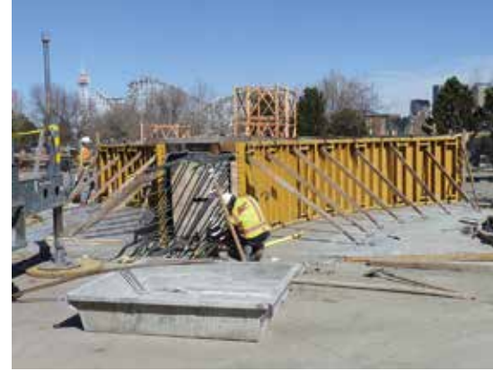
Precasting the interior piers.
