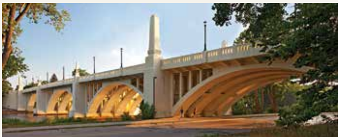
The concrete open spandrel arches of the Twyckenham Drive Bridge. Photo: Susan Fleck Photography.
