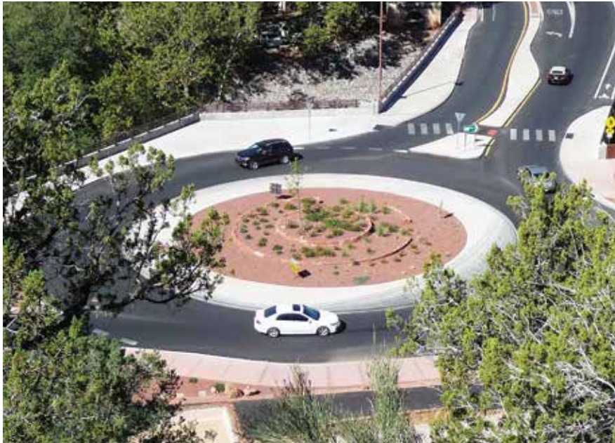
Completed SR 179 Oak Creek vehicular bridge. Photo: Steve Boschen.
