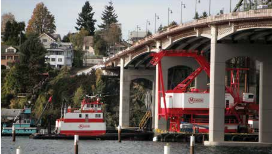
Structurally complete bridge with construction barges.
