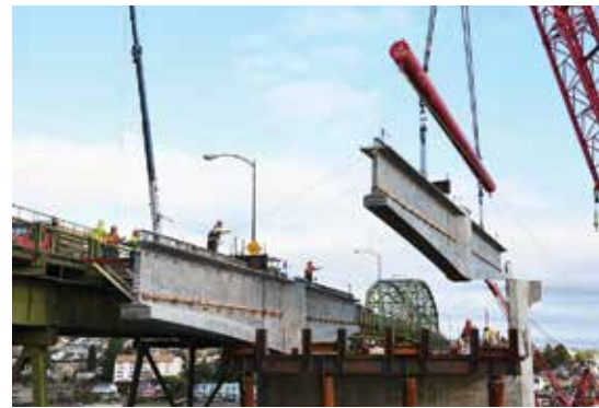
Hammerhead precast, prestressed concrete girders.
