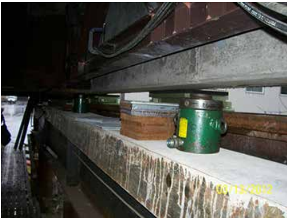
Hydraulic jacks are generally used to lift the bridge to install and remove rollers and install final bearings. All photos: Hilman Rollers.
