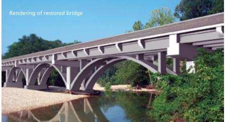
A precast concrete solution allowed the attractive arches on the Sinking Creek Bridge in the Ozark Scenic Riverways National Parkland to remain in place while appearing to support the bridge loads.
