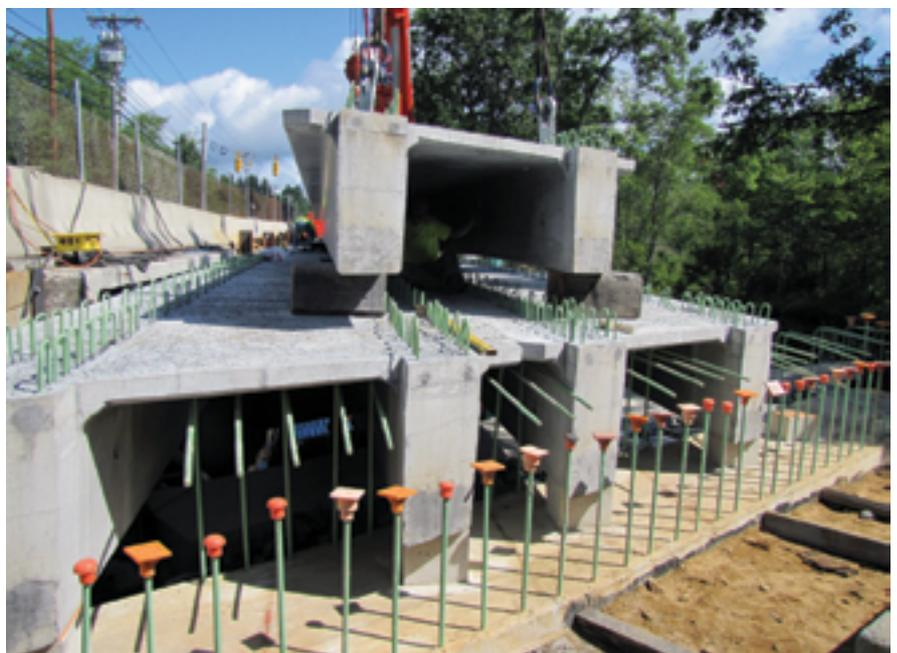
*The NEXT Beam, or Northeast Extreme Tee beam, developed by the PCI NE Technical Committee, is designed for rapid construction of bridges. This is the State Route 19 (Wales Road) Bridge in Brimfield, shown while still under construction in 2011. Photo: Massachusetts Department of Transportation.*
