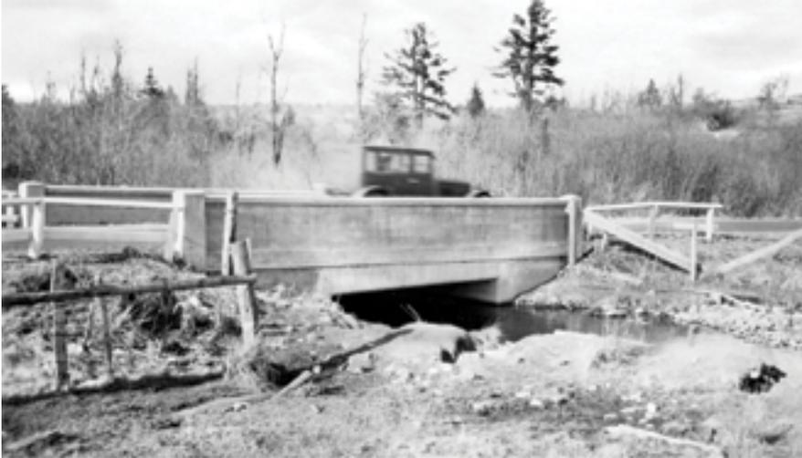
*A typical early reinforced concrete T-beam bridge built by the Massachusetts Highway Commission. This bridge, erected in 1909, is over Palmer Brook on what became U.S. 20 in the town of Becket. Photo: Massachusetts Department of Transportation Bridge Section Archives.*
