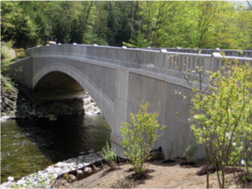
*The Sisk Bridge in Chester, carrying Old State Highway over the West Branch of the Westfield River was originally built in 1910 by the Massachusetts Highway Commission and rehabilitated in 2010. The original reinforced concrete arch is sandwiched between new arch extensions and spandrel walls, and carrying modern highway loads. Photo: CME Associates Inc.*
