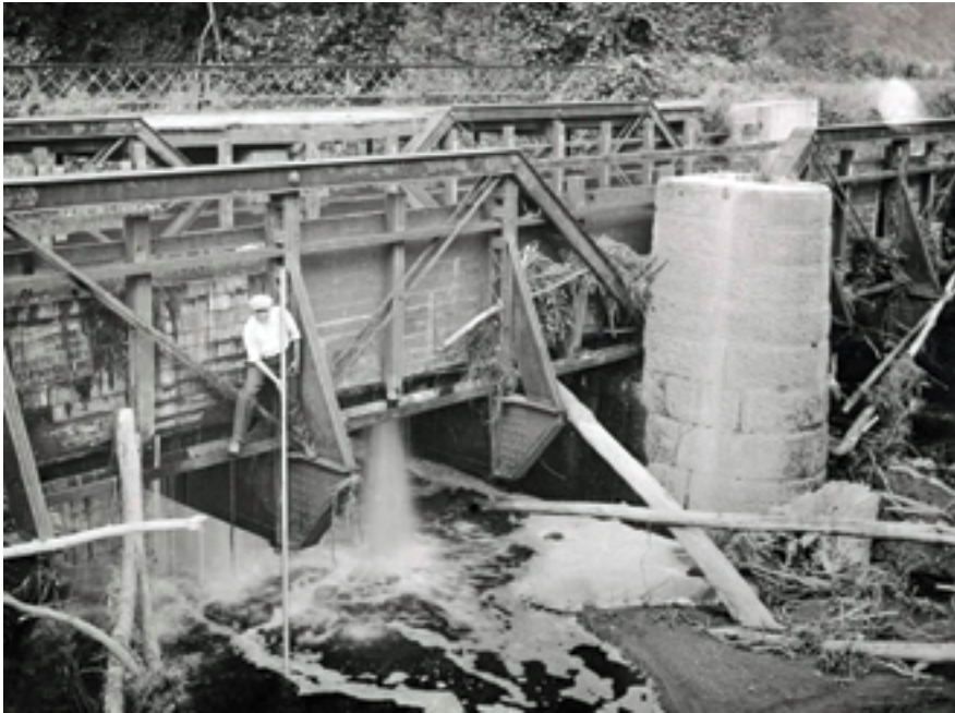
The 1905 aqueduct structure consisted of a two-span truss supporting a timber trough. Note the low freeboard to Tinkers Creek and significant debris accumulation. Photo: National Park Service.
