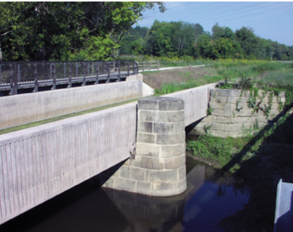
Elevation view of the new aqueduct and fully reconstructed masonry pier. Photo: Henry G. Russell Inc.
