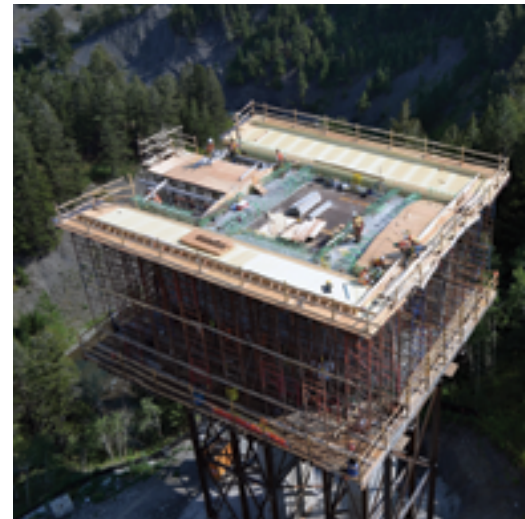
Overhead view of the Pier 2 pier table top slab forms.
