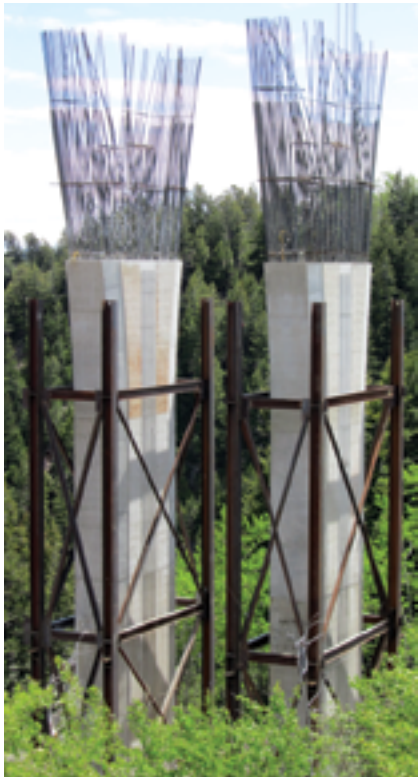
Pier 2 columns complete.
