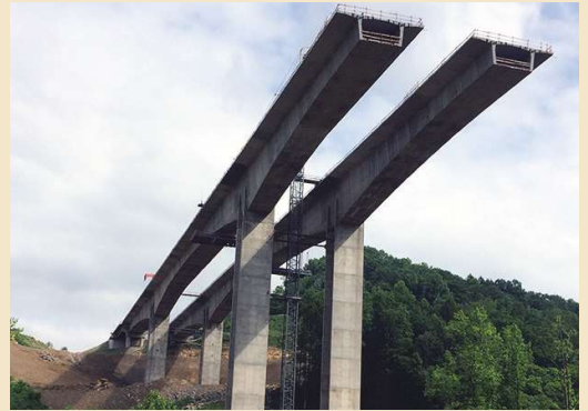
Two of the completed cantilevers highlight the curves of the structure.
