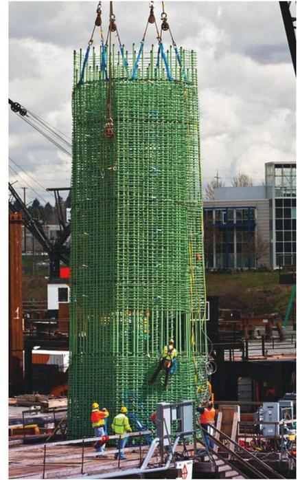
ASTM A775 reinforcing steel being placed for the Willamette River Bridge in Portland, Ore. Photo: Harris Rebar, Auburn.
