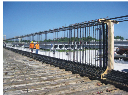
A 191-ft-long bridge girder used for the Cody Avenue Bridge in Okaloosa County, Fla., which used a straight strand profile during production. Photo: Dura-Stress Inc.
