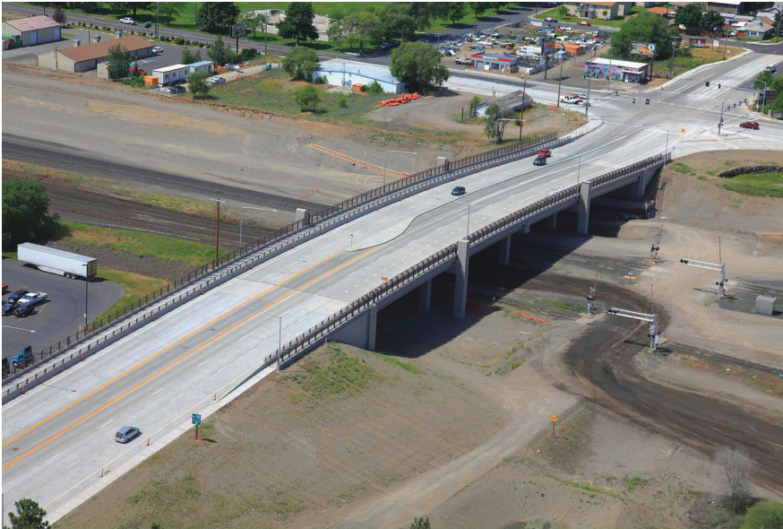
Aerial view of the Francis Avenue Bridge located in the north Spokane corridor in Washington state. All Photos: Washington State Department of Transportation Visual Engineering Resource Group (VERG).
