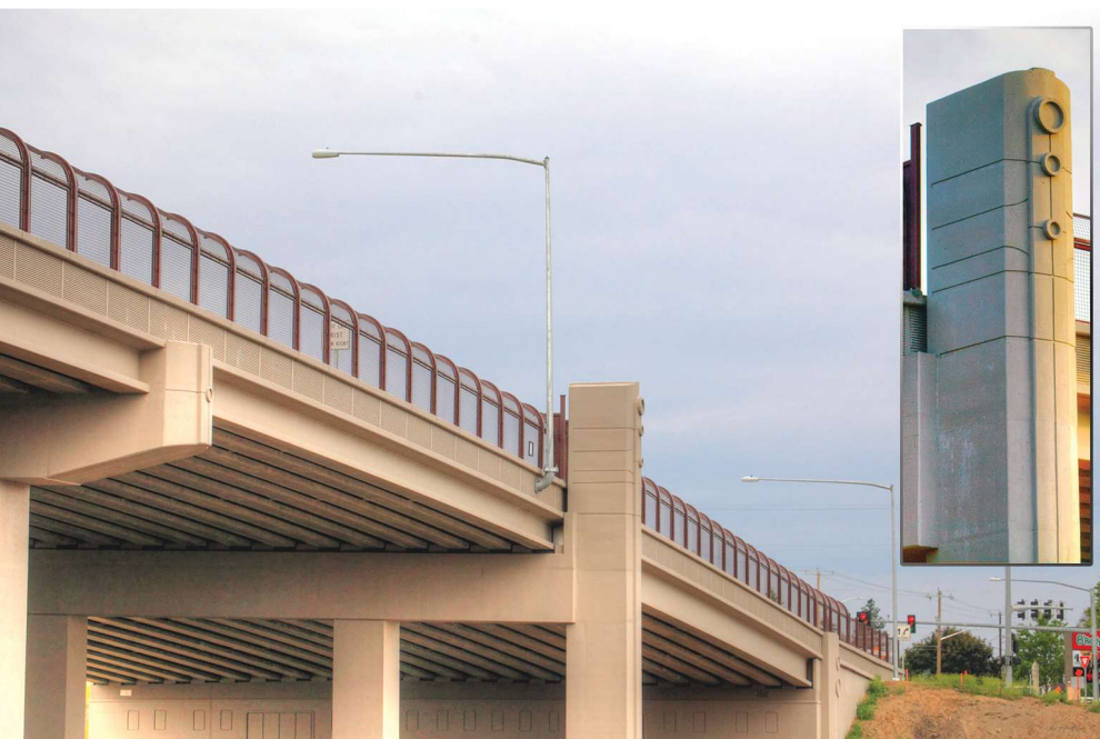
This photo shows how the different girder depths are obscured by the vivid railroad motif columns. Inset: Column design.
