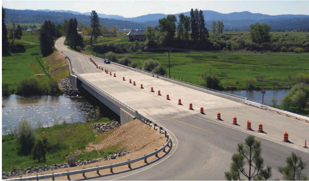
A single-span bridge was used as the replacement for the original five-span bridge. All Photos: Western Federal Lands.
