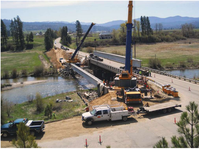
Setting girders for stage I (left) and stage II (right).
