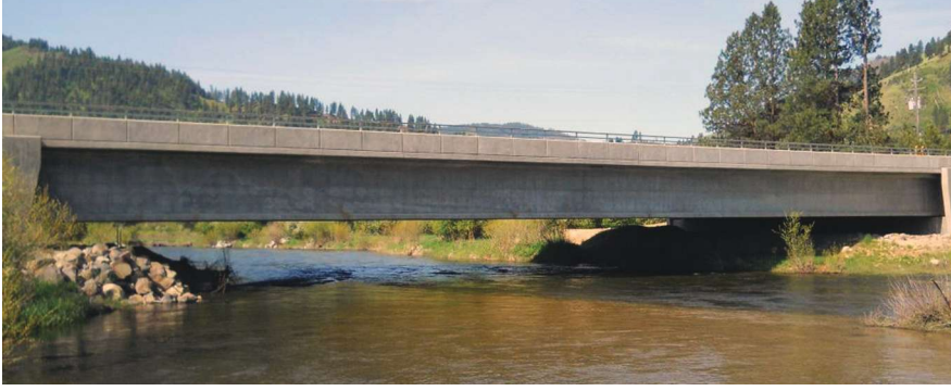
Upstream view of the bridge.
