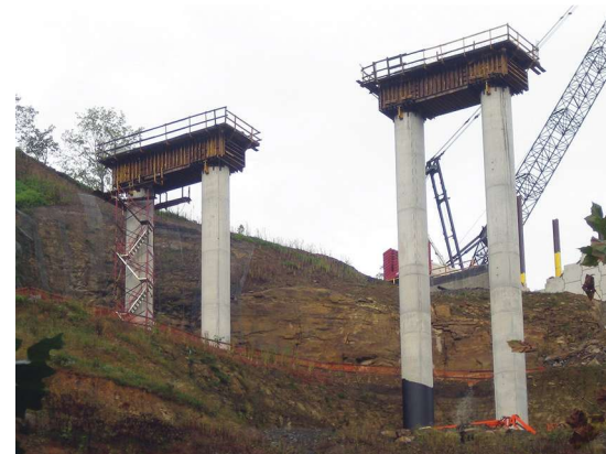
Piers 1 and 5 used two columns with a cap beam.
