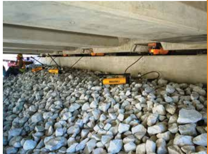
Lifting the bridge superstructure with pancake jacks to remove the rollers.
