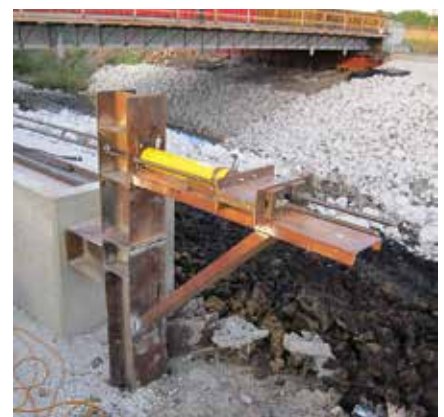
The jacking frame for pulling the prefabricated bridge superstructure into position.
