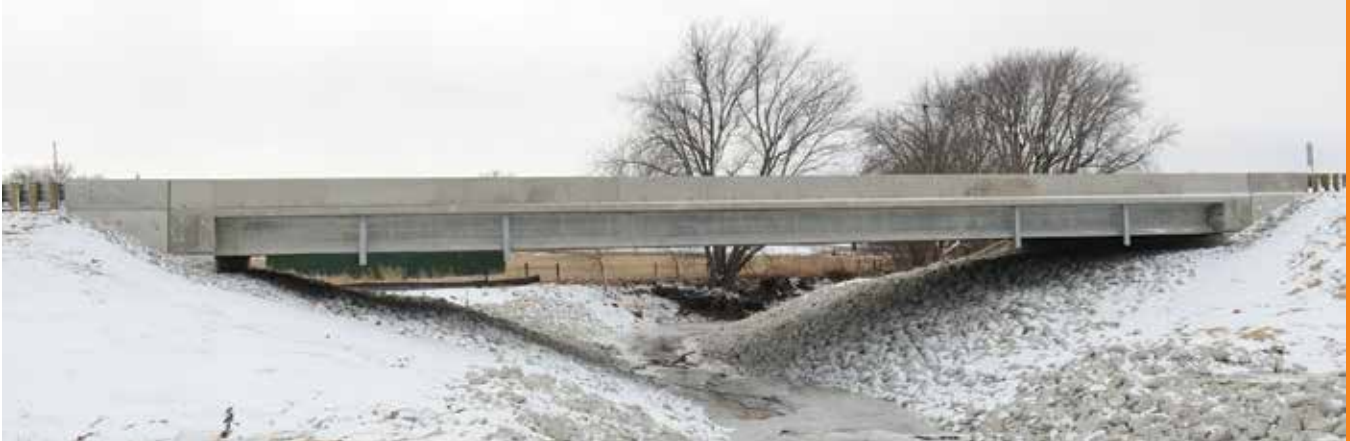
This photo shows the finished Massena Bridge after the lateral slide replacement. All photos: Iowa Department of Transportation.
