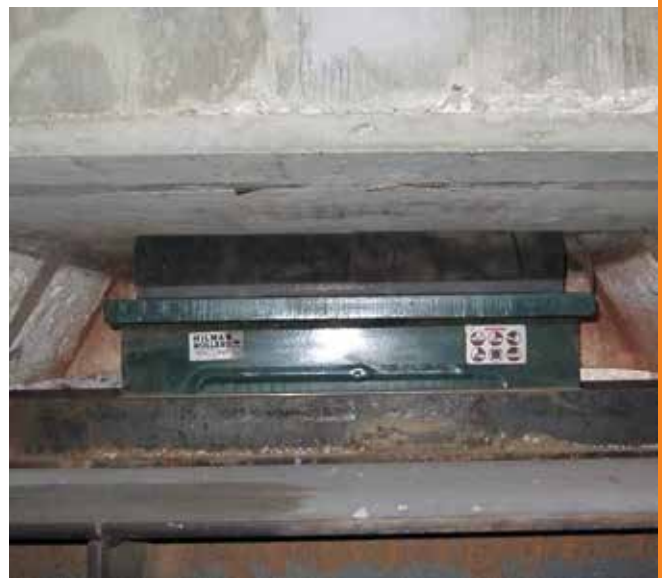
Roller in guide channel for rolling the prefabricated bridge superstructure.
