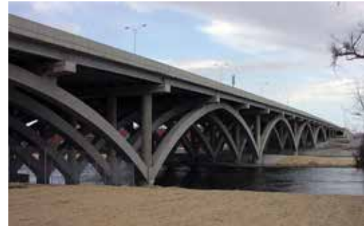
Reconstruction of the Fox River Bridge on the Reagan Memorial Tollway (I-88) was completed in 2009. Photo: Henry G. Russell Inc.
