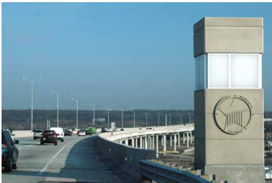
Traffic on the Des Plaines River Valley Bridge on the Veterans Memorial Tollway (I-355). Photo: Illinois Tollway.
