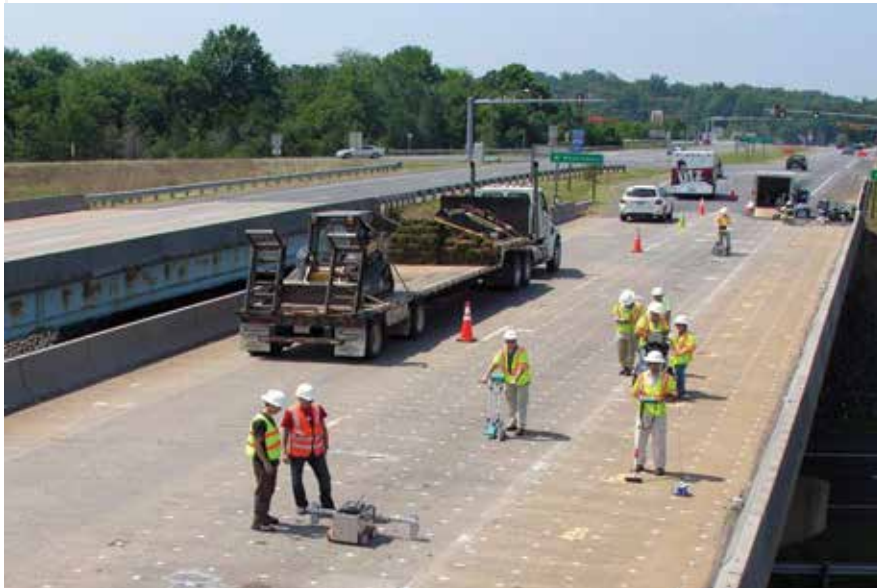
Various non-destructive evaluation technologies (impact echo, ground-penetrating radar, electrical resistivity, moisture scan, and half-cell potential) were deployed in the first pilot bridge to kick-off the Long-Term Bridge Performance Program. Photo: Federal Highway Administration.
