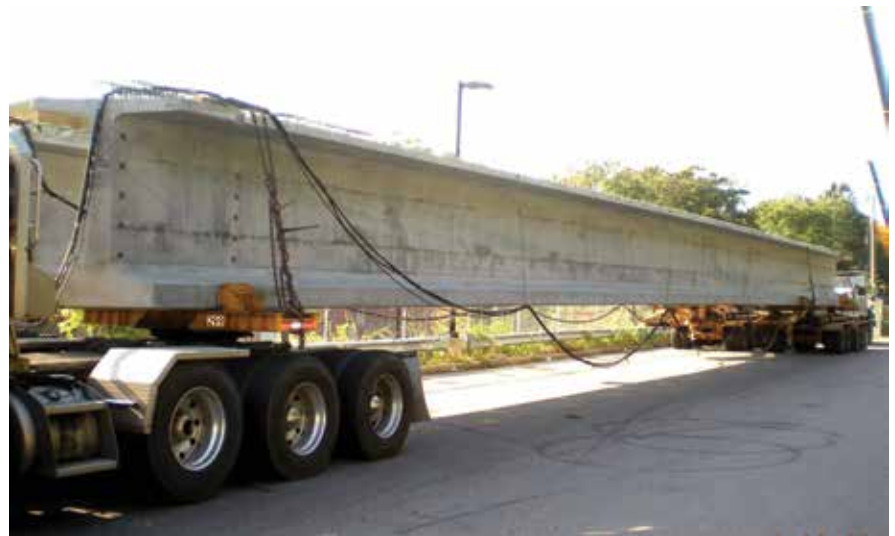
Precast concrete beams for the Fairmont Bridge Replacement were transported to the site by truck.
