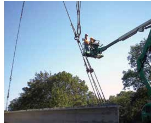
Crane load transfer during beam erection.
