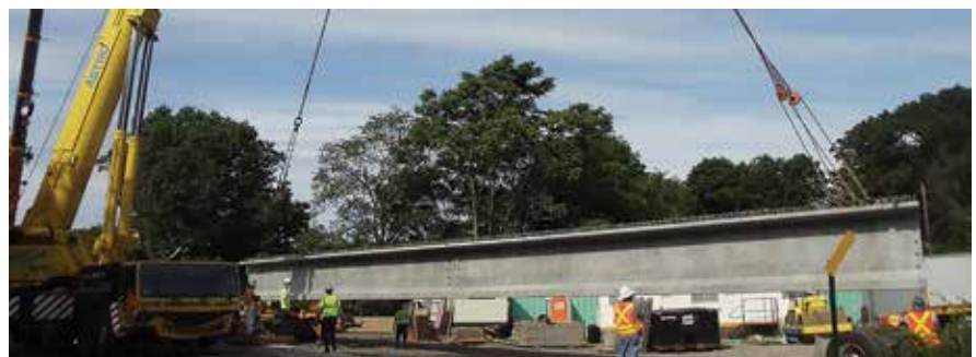
Elevation of one of the longest prestressed bulb-tee beams on bridge 2.
