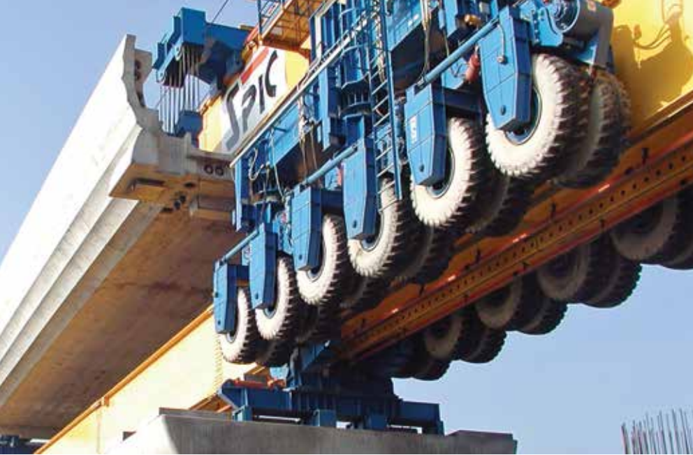
Portal carrier positioned for span lowering. Photo: Marco Rosignoli.
