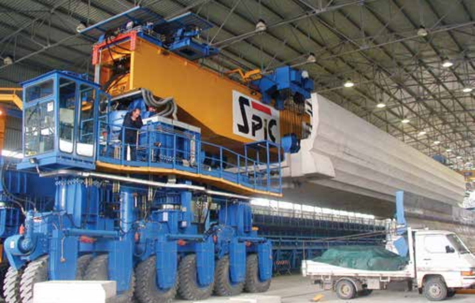
Span transfer to the storage platform with a portal carrier with pivoted tractors. Photo: Marco Rosignoli.
