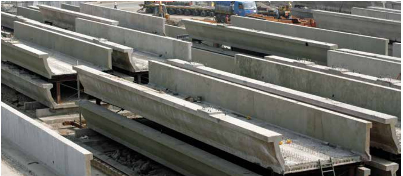
Span stacking on support frames. Photo: Systra.
