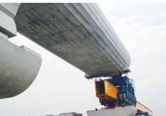
Repositioning of the underbridge. Photo: Marco Rosignoli.
