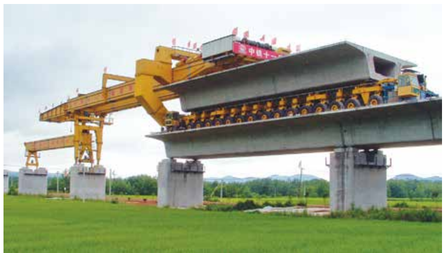
Tire trolley for 900-kip, single-track box girders. Photo: BWM.
