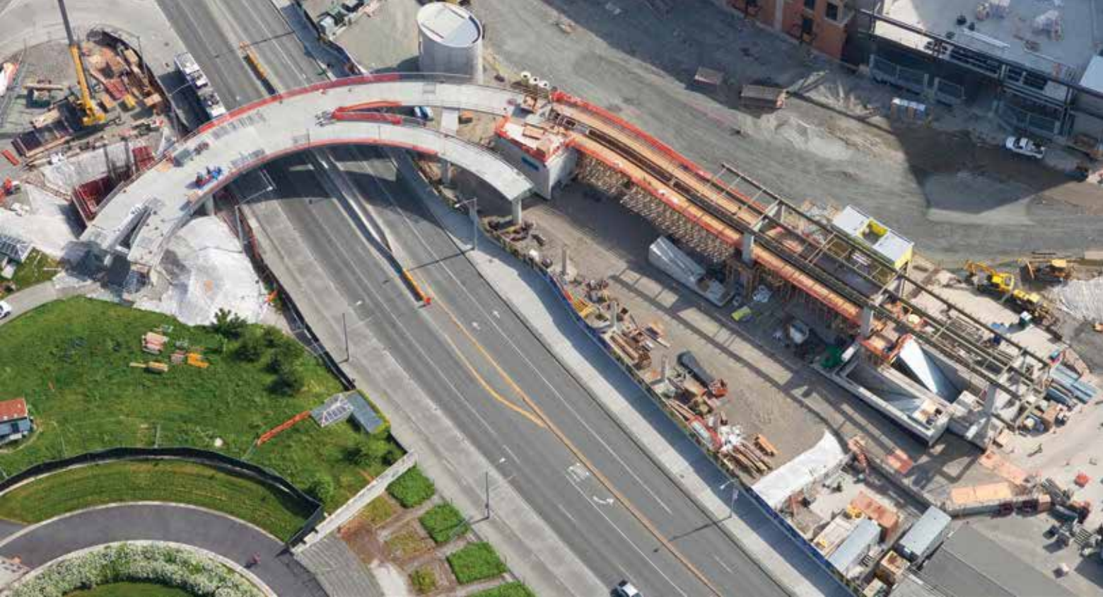
Montlake Triangle Pedestrian Bridge project. Photo: Sound Transit.
