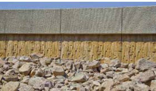
Concrete colors and textures complement natural riprap slope protection.
