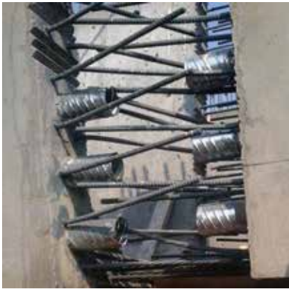
Close up of the splice between precast concrete girder segments.
