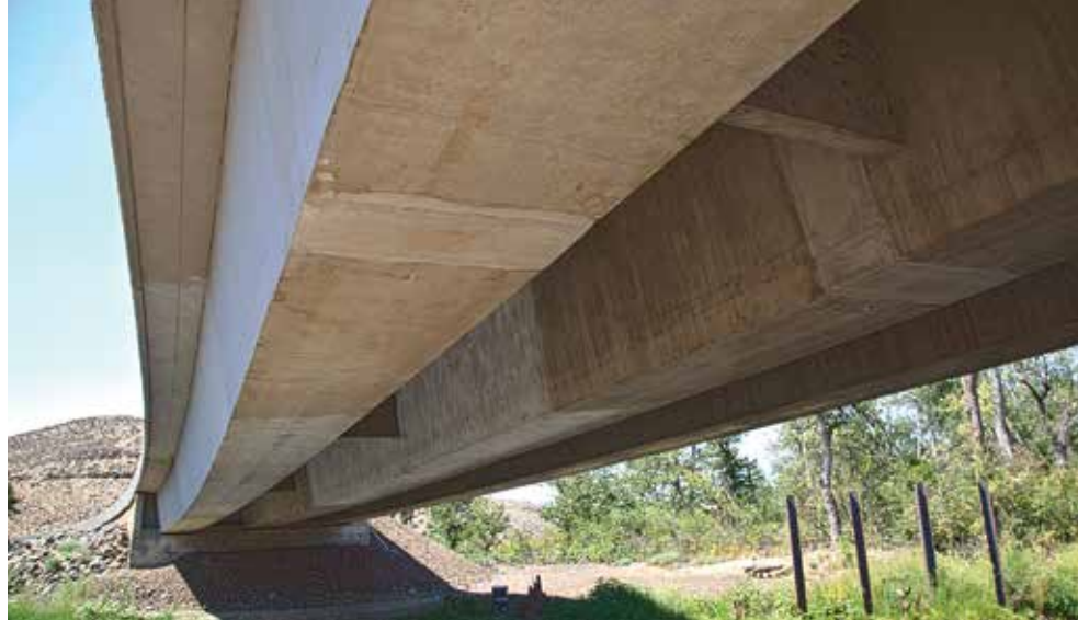
Curved trapezoidal girders showing closure concrete placements and diaphragms.
