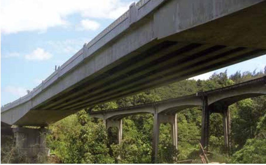
Kealakaha Stream Bridge with existing bridge in background.
