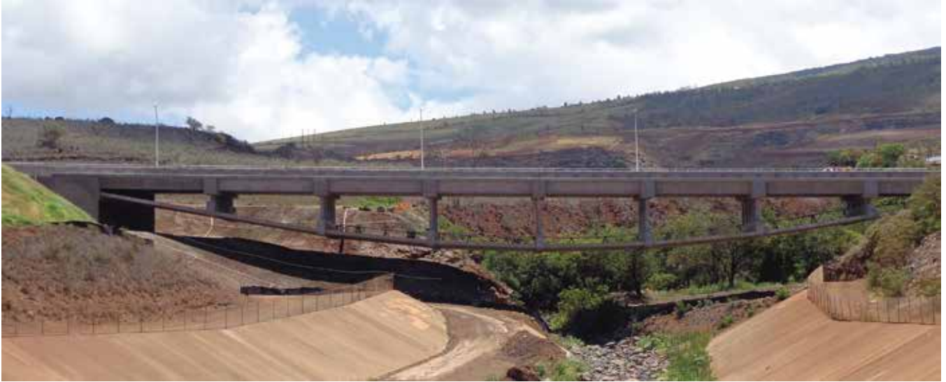
Kahoma Stream Bridge. All photos: KSF Inc.
