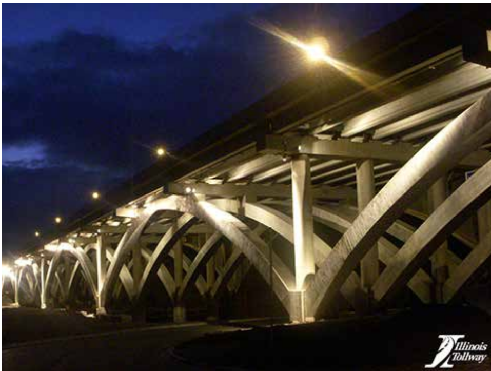
Reconstruction of the Fox River Bridge on the Reagan Memorial Tollway (I-88) was completed in 2009.
