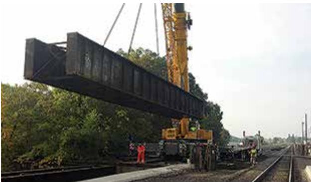
Demolition of old steel structure.
