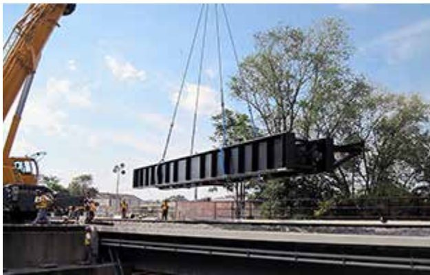
Elevation of prefabricated steel plate girder, picked up by crane over the bridge at mile
