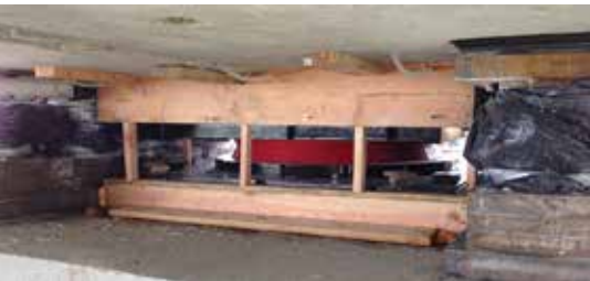
Newly installed pier disk bearing with pressure grouting formwork.
