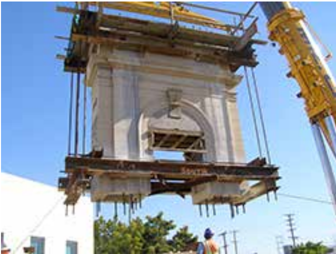
Moving the triumphal arch. Photo: Atkins North America.
