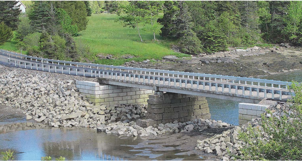
Bridge open for traffic. All photos: Town of North Haven, Maine.
