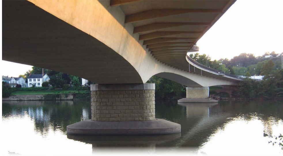
Putnam Bridge piers 1 and 2 south elevation. Photo: Julia David, Barr & Prevost.
