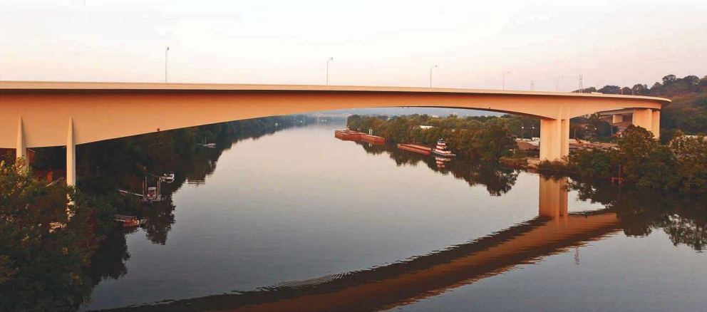
The combination of prestressed concrete and segmental construction allowed a main span length of 760 ft for the Kanawha River Bridge, W.Va. Photo: T.Y. Lin International.
