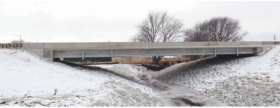
The concept of accelerated bridge construction is changing the way that bridges are replaced, such as the Massena Bridge in Iowa. Photo: Iowa Department of Transportation.
