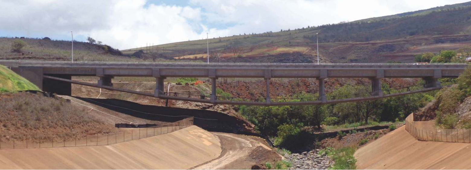
Elevation view of Kahoma Uka Bridge. Photo: Chad Nikaido.
