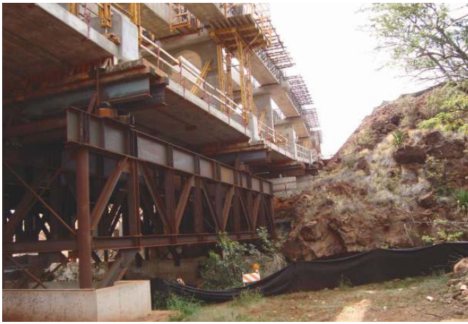
Falsework truss installed to span Kahoma Stream. Photo: Eric Matsumoto.
